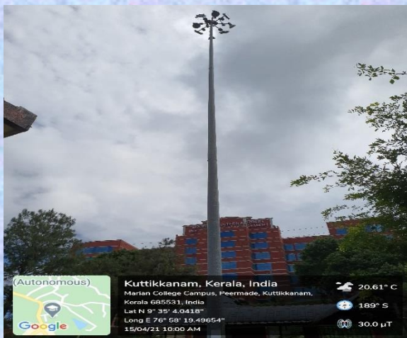
High Mast Light with timer
