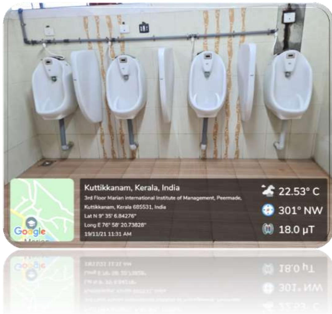
Sensor Based Urinals for saving water
