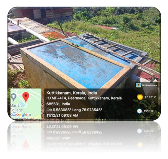
The Bar Screen Chamber of sewage treatment plant for separating plastic and other non-decomposable materials from the incoming waste water
