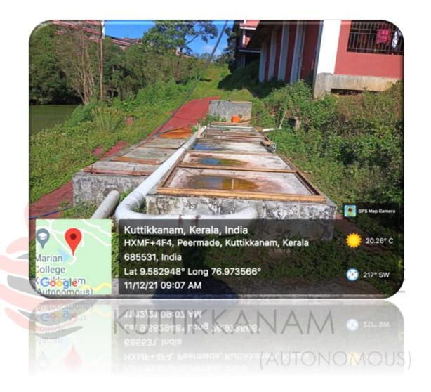
The Grit Chambers slow down the flow of wastewater for separating the floating solids
