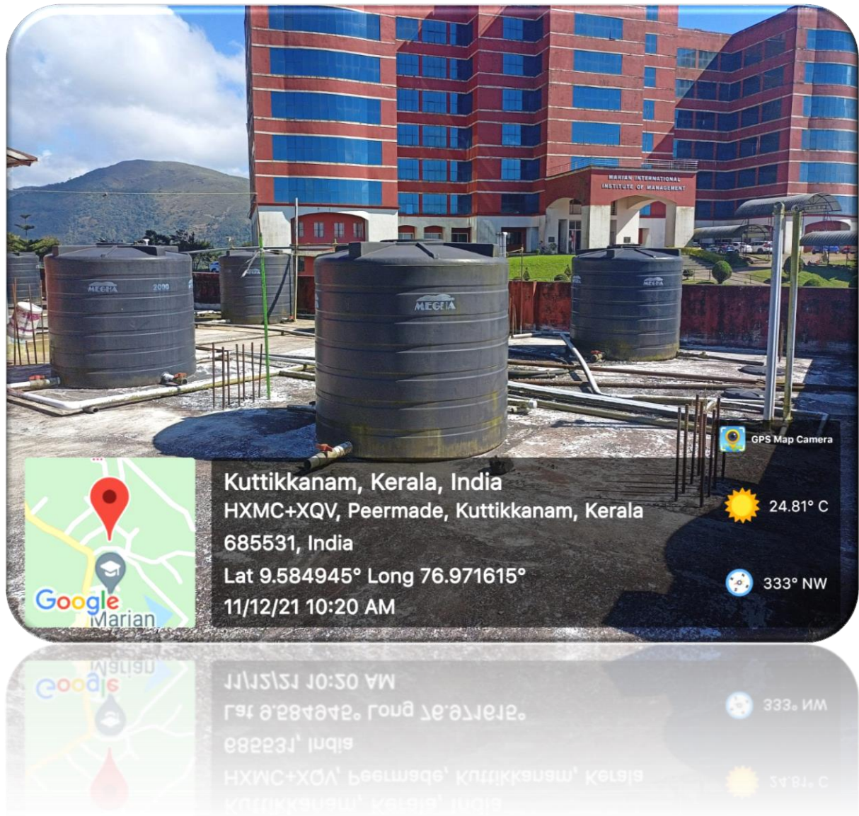
The water containers and the distribution pipes on the top of staff quarters
