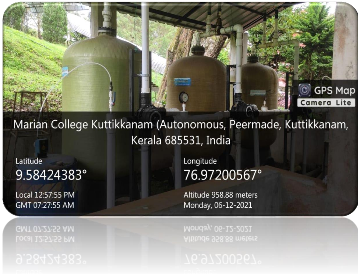
Water filtration unit and its distribution system near the reservoir 2
