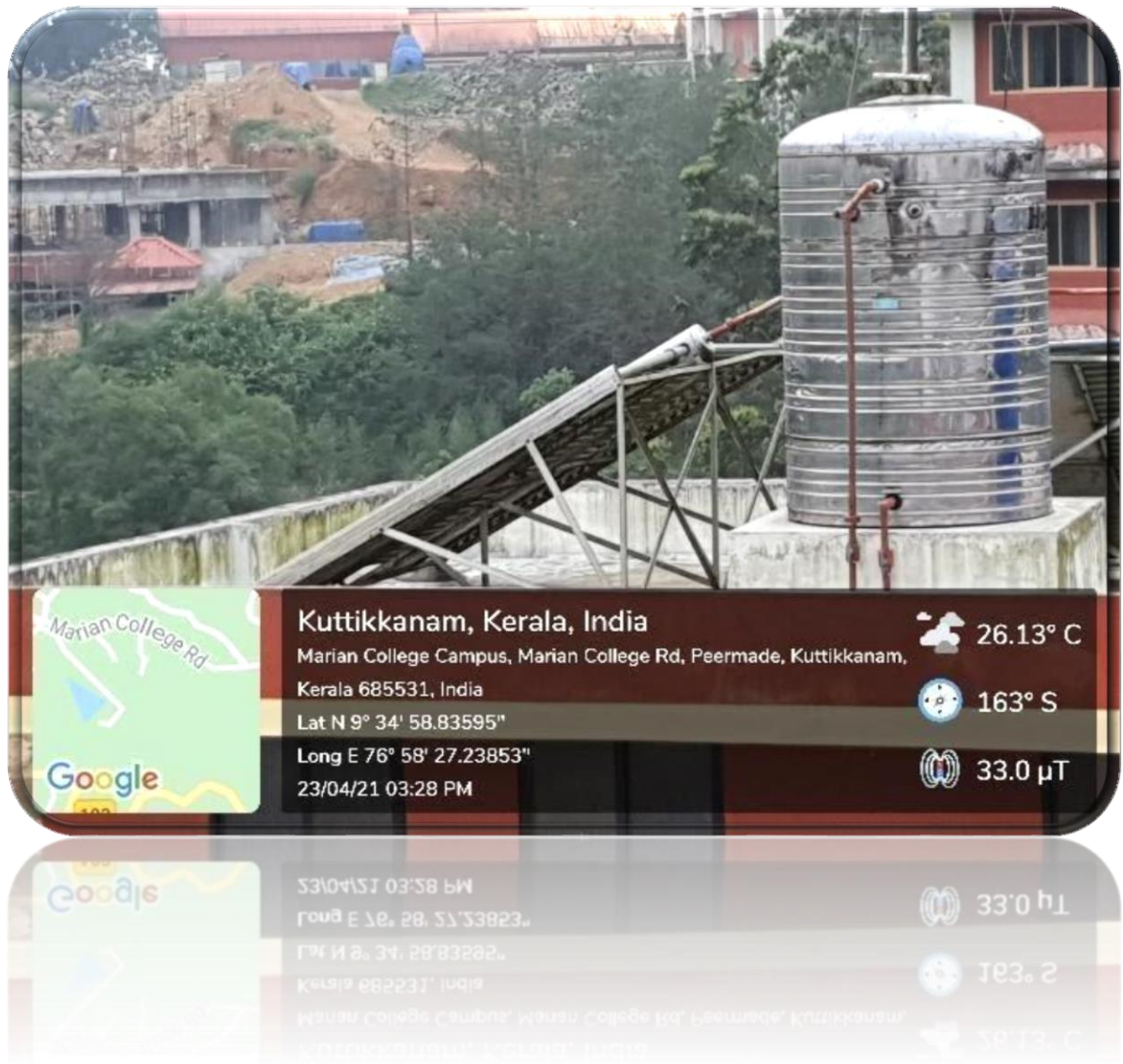
The solar panel, water container and its distribution system for hot water in the hostels
