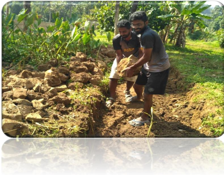
e Preparation of Water Harvesting Pits
